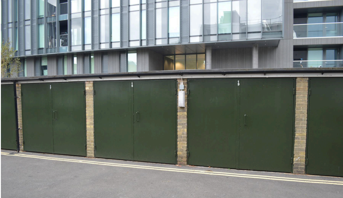
SPRAY PAINTED GARAGE DOORS FITTED WITH DEAD LOCK, WRAYBURN PROJECT
